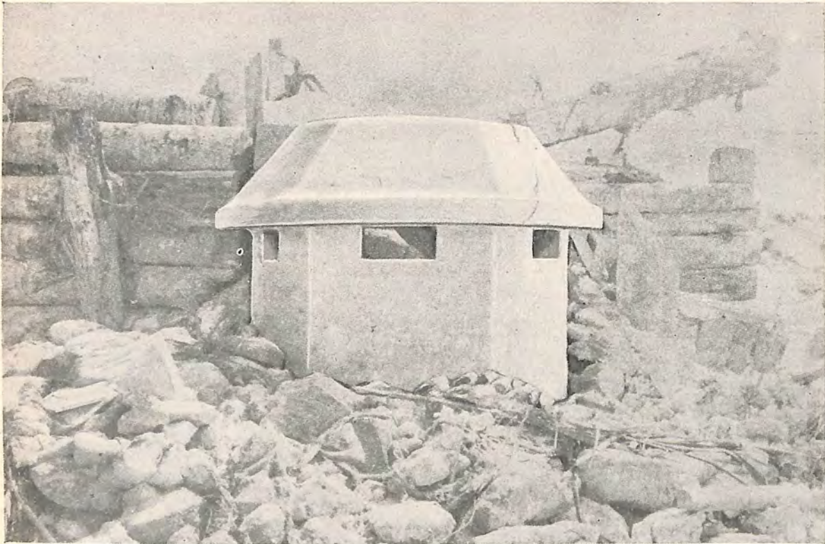
Figure 146. A concrete pillbox.
